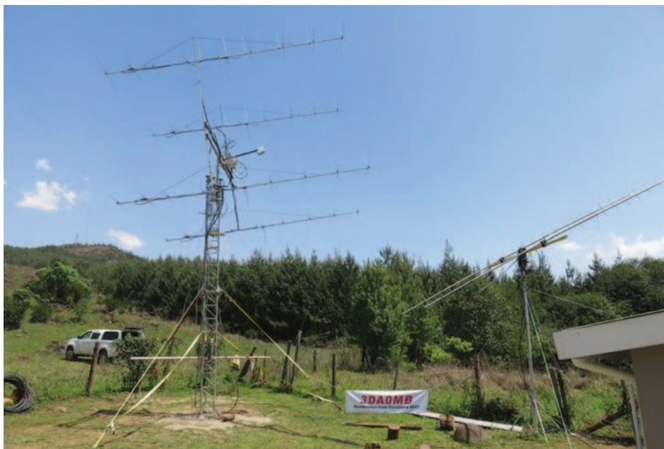
The 3DA0MB antenna farm in Swaziland. An excellent EME (moonbounce) signal.
