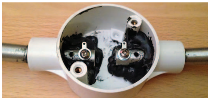
PHOTO 3: Alternative loop termination using a plastic conduit box.
